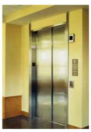
STANDBY Smoke Guard is contained in a metal housing and mounted above the lift door on the lobby side of the lift shaft.
