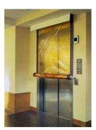
ALARM Smoke Guard automatically deploys when smoke is detected by the smoke detector in front of the lift door or on general alarm.
