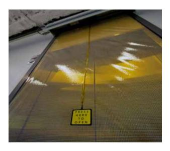
Smoke (Air) leakage of less than 0.3m3/min per m2 of door opening @ 200°C when tested in accordance with AS1530.7, providing the lowest smoke leakage available for any smoke containment screen in the world.
