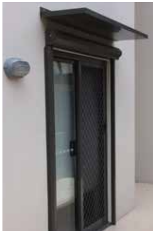
Typical head box section
