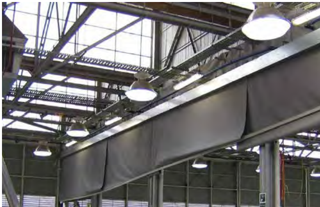
| Overlapped systems often lead to noncompliant and unsafe buildings.
