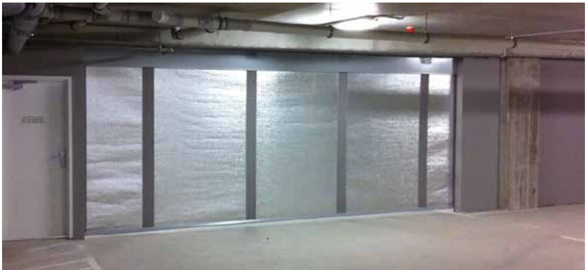
| Fibershield ULR being used in Australia to fire separate a basement car park. Fibershield ULR also provides smoke separation, a feature not offered by other methods.
