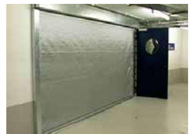
Fiberseal FS fire and smoke containment screen used to separate a carpark from a shopping centre to upgrade existing glazing system. The system has commenced deployment. See full deployment below.
