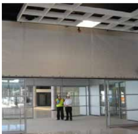
Fibershield 4 protecting an existing installation of non-fire rated glazing
